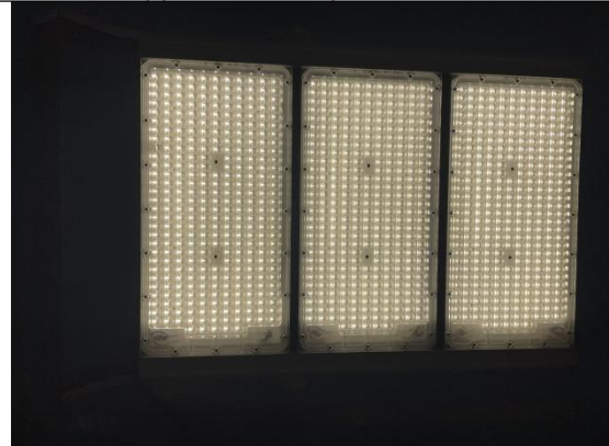
Light up inspection
