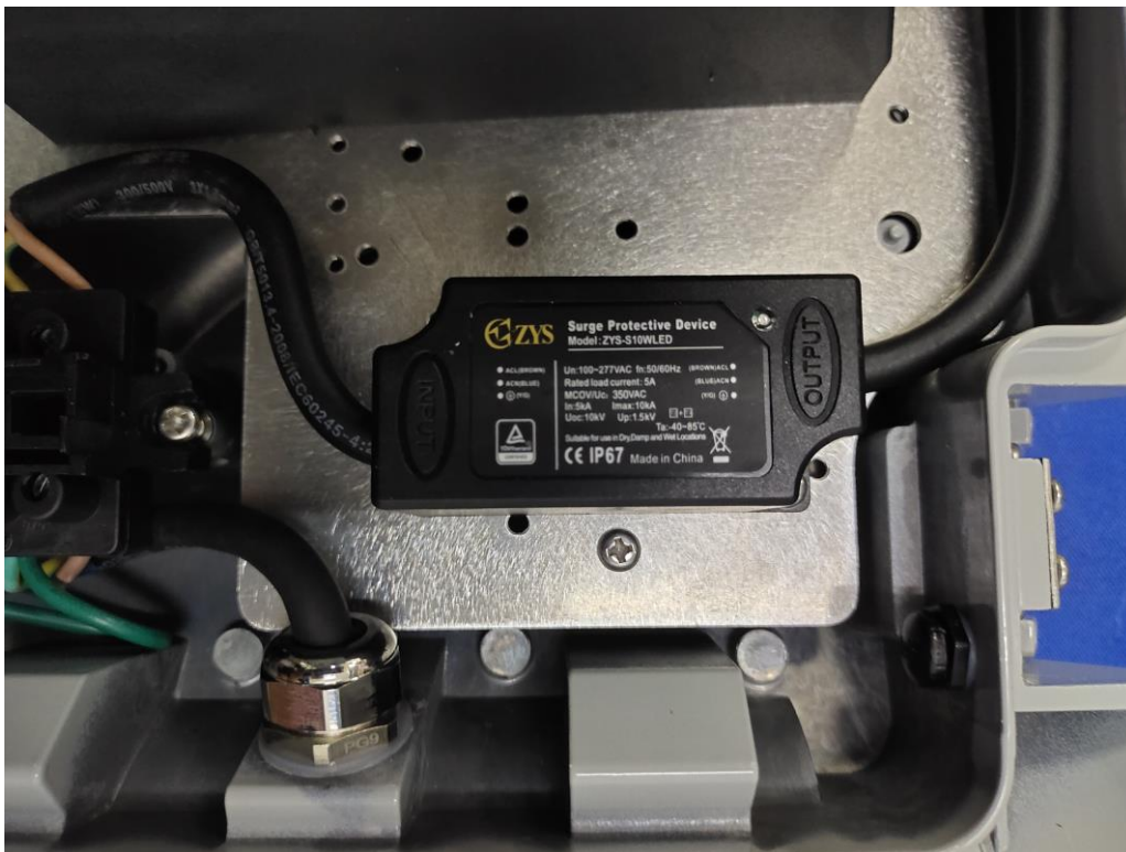
Picture 5. Surge protective device view
