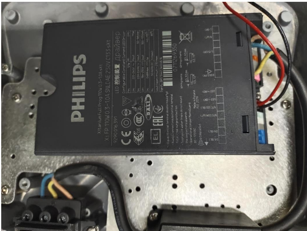
Picture 4. LED driver view for all models
